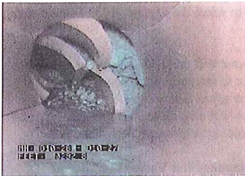
CRUSHED PIPE
